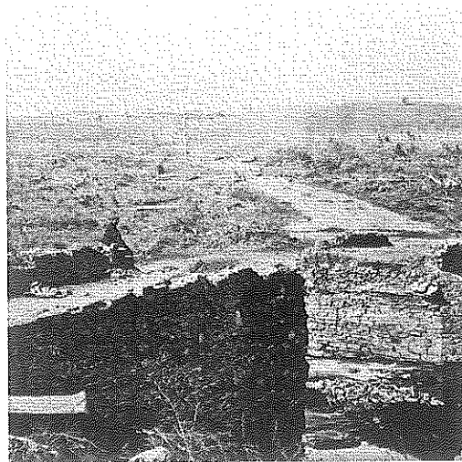
Broken bridge over Bull Run Outside Manassas, VA
